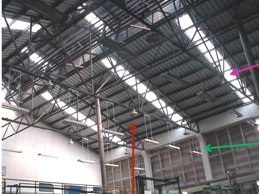
Mercury Vapor Lamp
