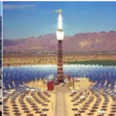
Concentrating solar power tower – courtesy Sandia National Laboratories
