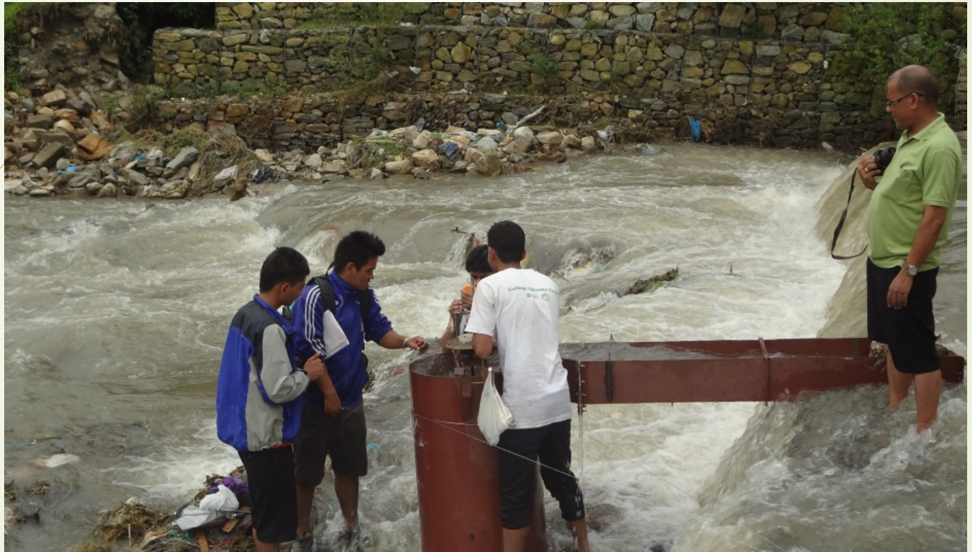
Figure : Installation in Manohara River, Bagmati, Nepal
