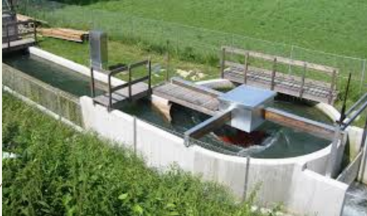
Figure : First Power Plant
