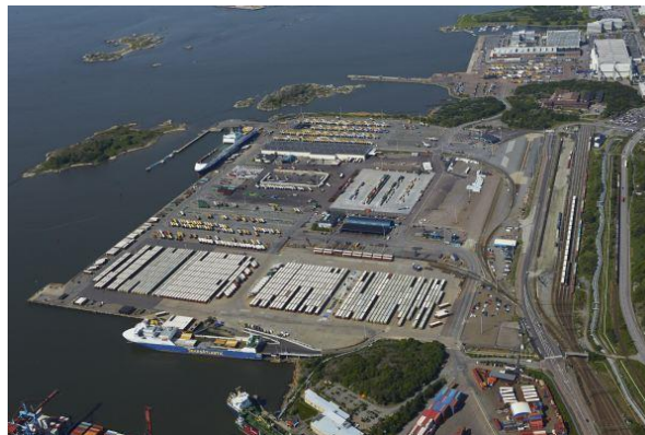
Port of Gothenburg
