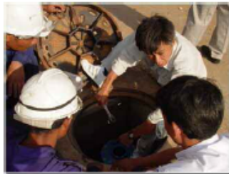
Water supply project at Phnom Penh
